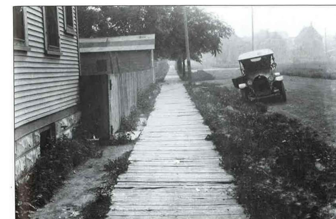
WOODEN SIDEWALKS, 1919. The older sections of West Allis were lined with wooden sidewalks. This walkway in William Shenners subdivision, east of South Sixtieth Street and north of National Avenue, shows the unevenness and problems of a wood sidewalk. In the 1920s, the city gave homeowners a tax incentive to repair the sidewalks. Maintenance was an ongoing issue and concrete sidewalks replaced many of them in the 1930s.
